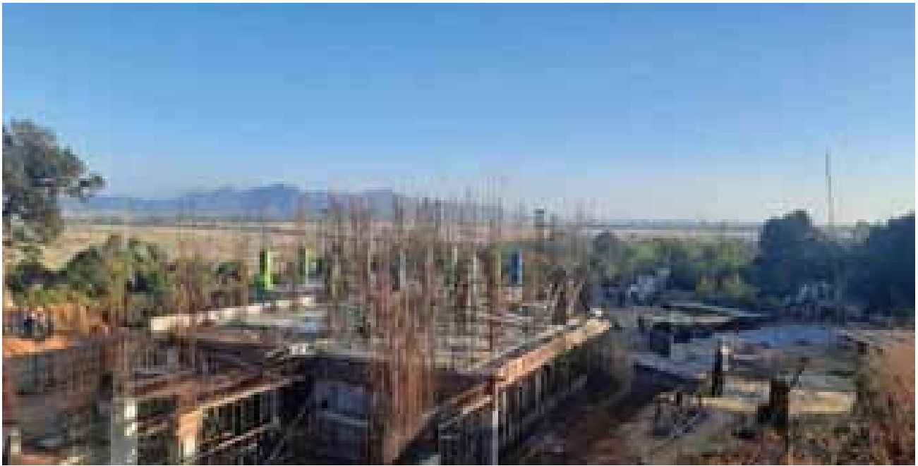
On going construction of new campus
